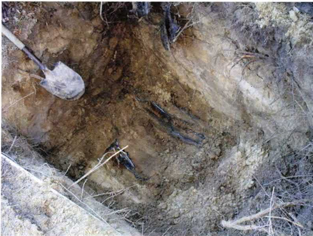
Picture 2: UST 926Albacore excavation.
